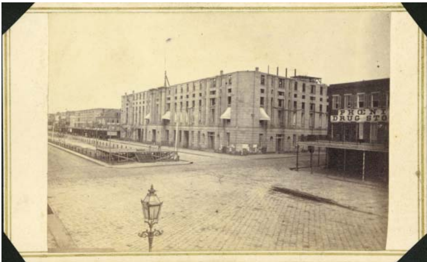
Custom House, Canal and Levee Street. Construction began on the New Orleans Custom House in 1848 but was not completed until after the American Civil War. Interestingly, images published in Harper's Weekly Magazine show the building completed. The blue 2 cent tax stamp on the verso of this image was cancelled, 16/9/1864. Marshall Dunham Photographic Album (Mss. 32410059), Louisiana and Lower Mississippi Valley Collections, LSU Libraries, Baton Rouge, Louisiana, USA.
