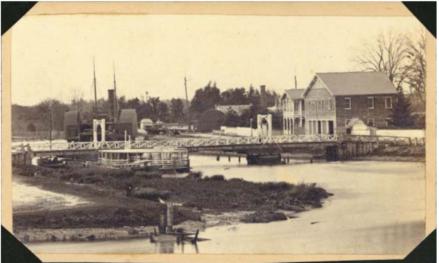
Bayou Bridge Station. This bridge crosses Bayou Saint John near the present day intersection of Esplanade and City Park Boulevard. A canal leading into the heart of the city connects to the bayou at this point providing access to the city from Lake Ponchartrain. Note the 2 ironclads moored above the bridge in Bayou Saint John. Marshall Dunham Photographic Album (Mss. 32410042), Louisiana and Lower Mississippi Valley Collections, LSU Libraries, Baton Rouge, Louisiana, USA. Mark Martin's remarks about this amazing album begin on p. 17.
