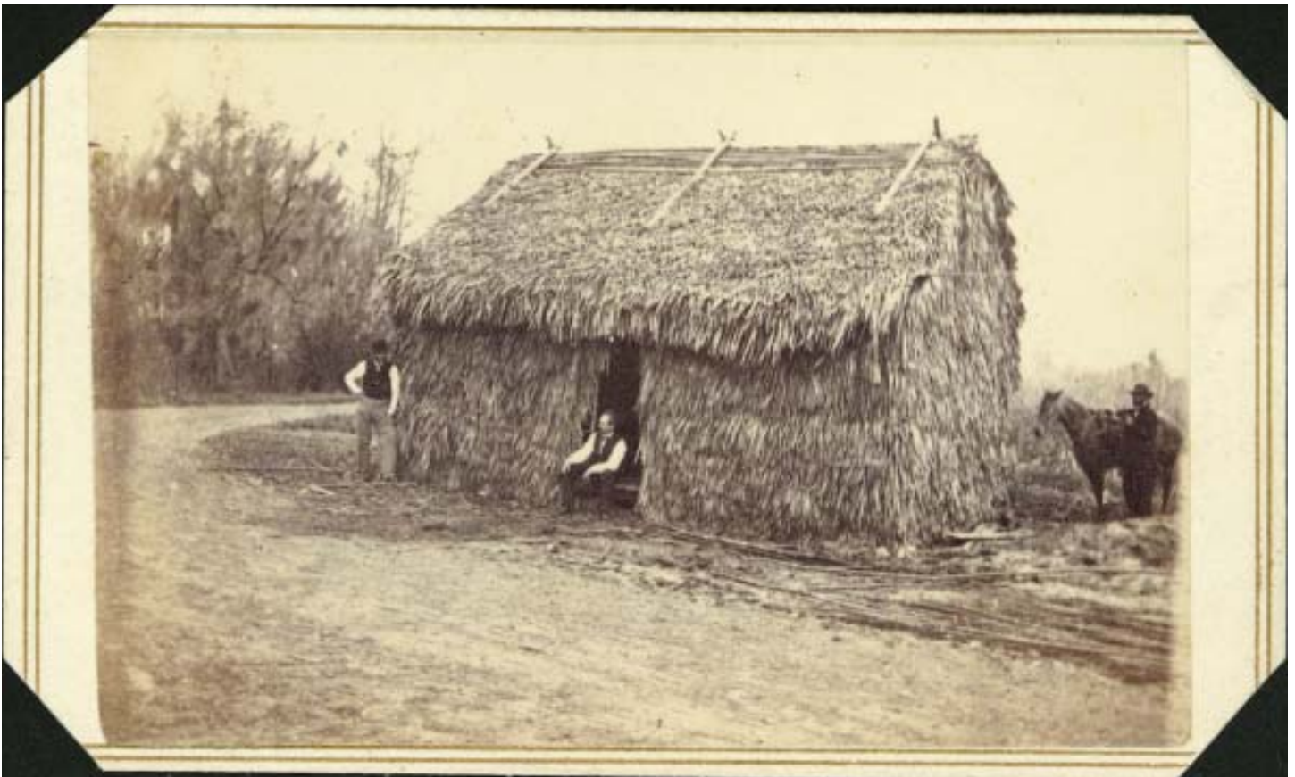
Thatched hut - Houma. Not much else is known about this image. Information about who the people are and why this cabin was built is lost. It does, however, give us an example of temporary building construction methods using materials at hand as the thatch is either palm or palmetto fronds. Marshall Dunham Photographic Album (Ms. 3241084), Louisiana and Lower Mississippi Valley Collections, LSU Libraries, Baton Rouge, Louisiana, USA. Mark Martin's remarks about this amazing album begin on p. 17.
