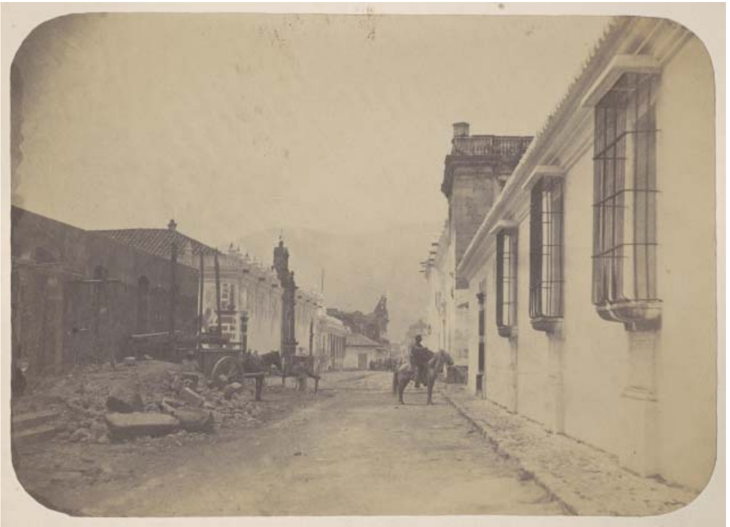
J. H. Fitzgibbon. Street of San Lazaro. Antigua, Guatemala [Showing the destruction caused by an 18th century earthquake], 1858. Salt print from wet collodion negative. John Melmoth Dow papers, #2765. Division of Rare and Manuscript Collections, Cornell University Library.
